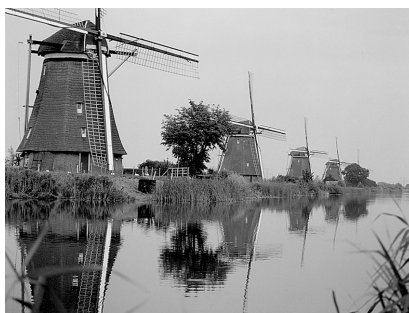
Figure 3.1: Drainage by series of windmills (Source: Rijkswaterstaat)
