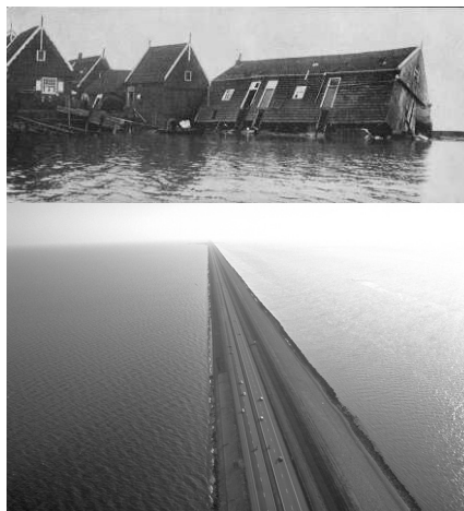
Figure 3.2: The 1916 flood damage, especially in areas bordering the Zuiderzee area (top), triggered the closure of the Zuiderzee by the 'Afsluitdijk' (bottom) (Source: Rijkswaterstaat)
