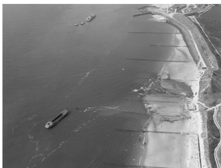
Figure 3.6: Example of a nourishment scheme (Source: Rijkswaterstaat)
