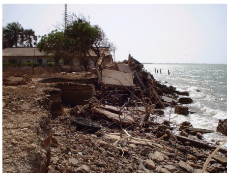
Figure 2.7: Coastal erosion threatening property
